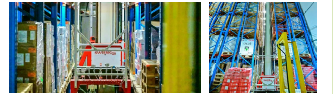
Swisslog Automated Warehousing System
